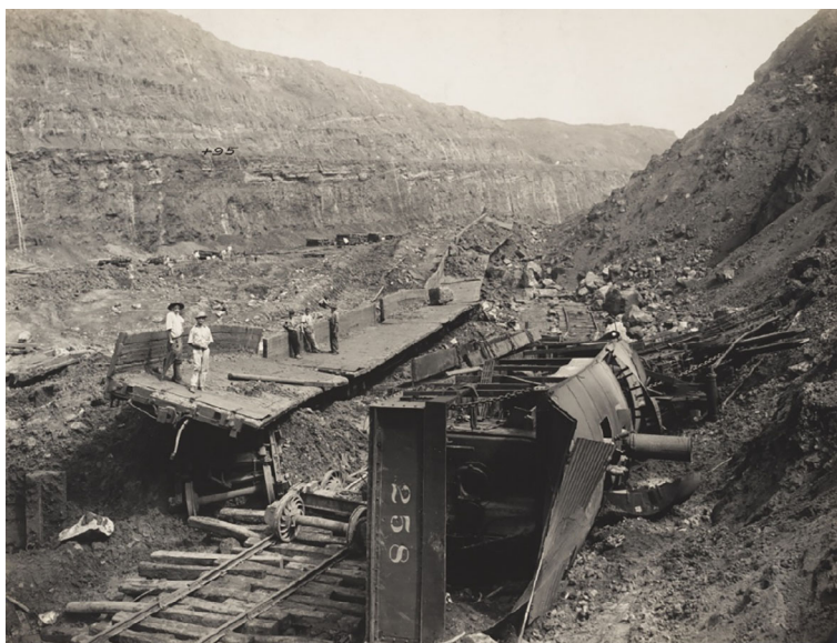
FIGURE 1 Pro-active geoengineering experiencing limits of controlling nature: landslides at the construction site of the Panama Canal in May 1913. Courtesy of The Linda Hall Library of Science, Engineering & Technology; LHL, A. B. Nichols Collection, Notebook Vol. 48B, p. 65
